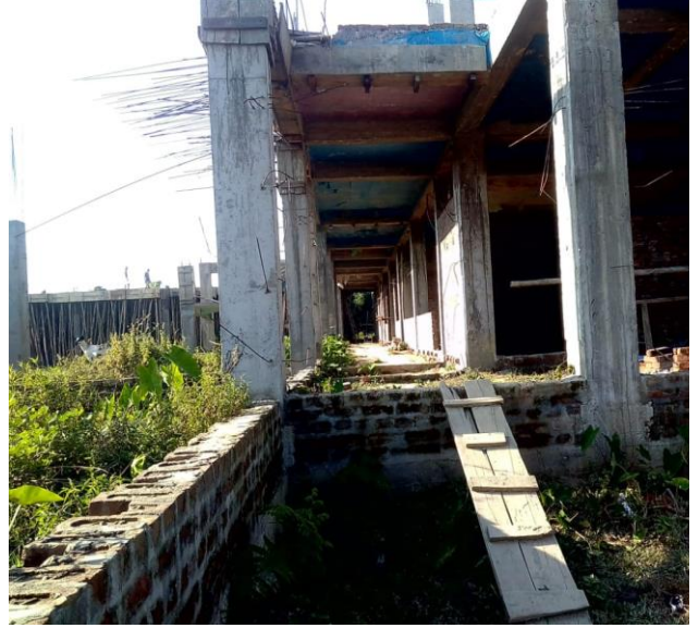
Govt. MDC- Kakopathar, Tinsukia (Construction works are going on)
