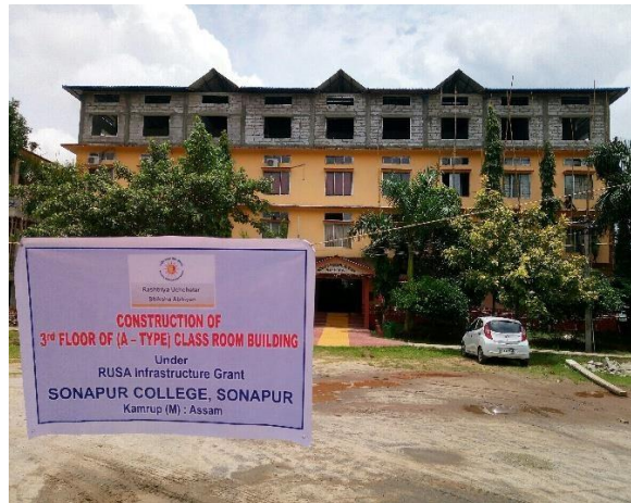
Construction of Classroom Building, Sonapur College
