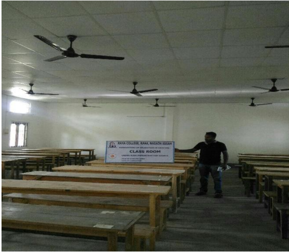
Renovation of Classroom, Raha College
