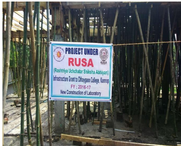
New Construction of Laboratory Building Chhaygaon College
