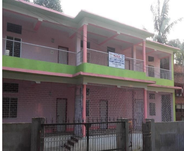
Construction of Boy's Common Room and Students Union Society Hall, Pandu College
