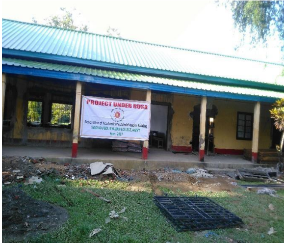
Renovation of Academic Building, SPP College
