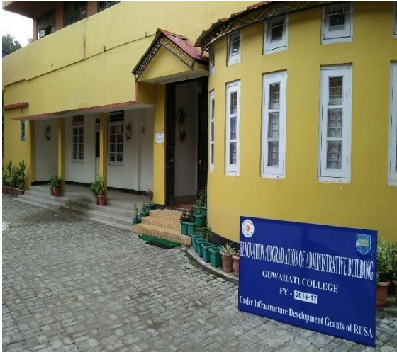
Renovation/Upgradation of Administrative Building, Guwahati College
