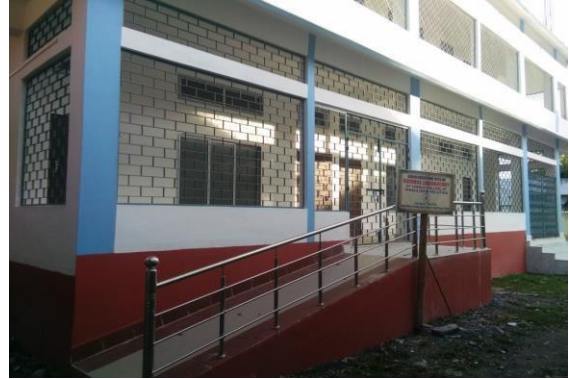
Construction of Science Laboratory of Tangla College
