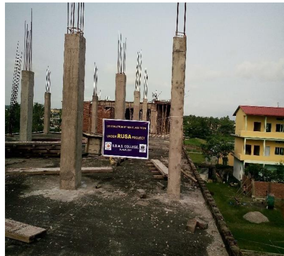
New Construction, SBMS College
