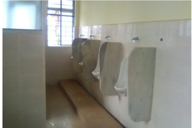
Gents toilet at department of Statistics
