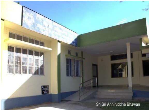
Renovation of Aniruddha Bhawan with Director's room and Library (Phase-II)
