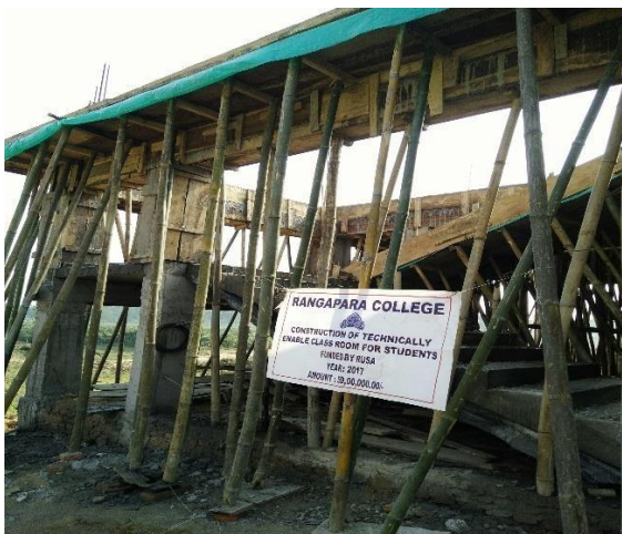
Construction of Technically Enabled Classroom, Rangapara College
