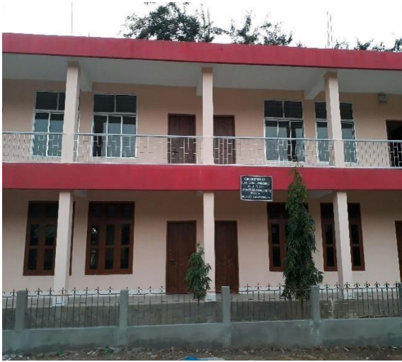
Construction of Classroom, Laboratory & Girls' Toilet, Nanda Nath Saikia College
