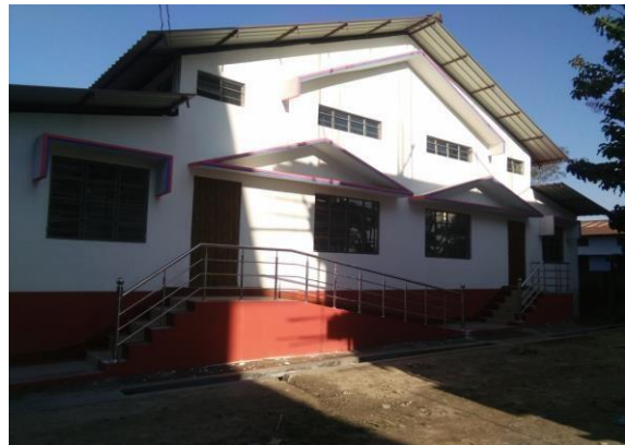
Extension of Auditorium Hall- Tangla College
