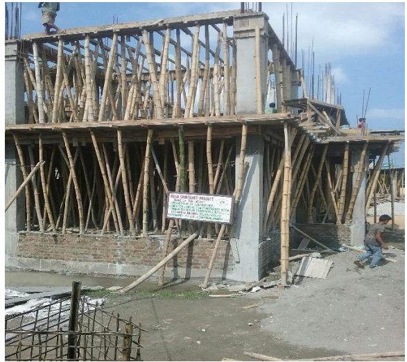
Construction Work, Puthimari College
