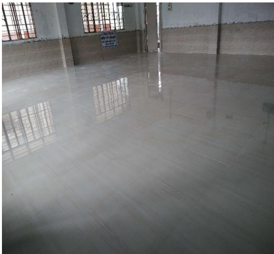
Renovation work, S.B. Deorah College
