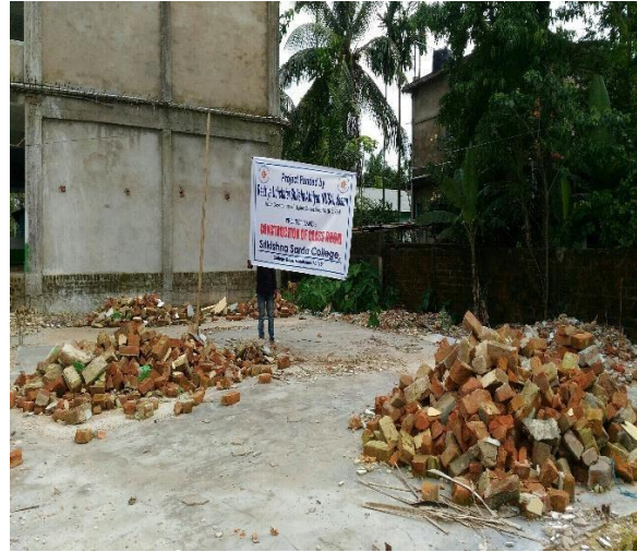
Construction of Classroom, SS College
