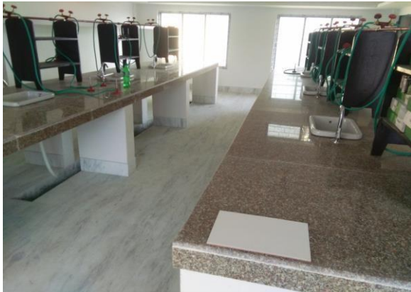
Construction of Science Laboratory of Tangla College
