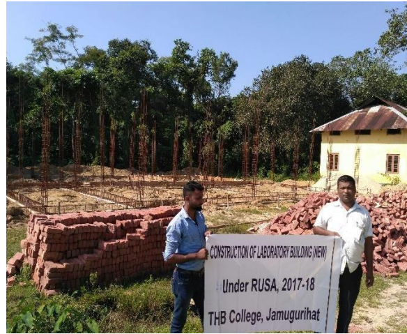
Construction of Laboratory Building, THB College
