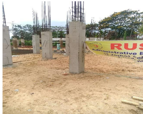
Construction of Administrative Building, Jorhat College
