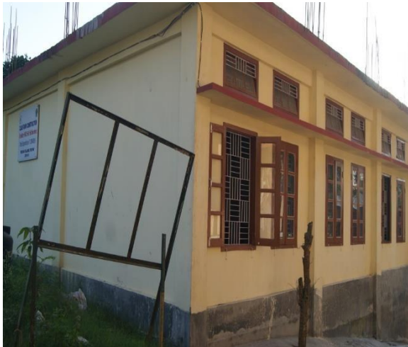
Construction of Classroom, Tezpur College
