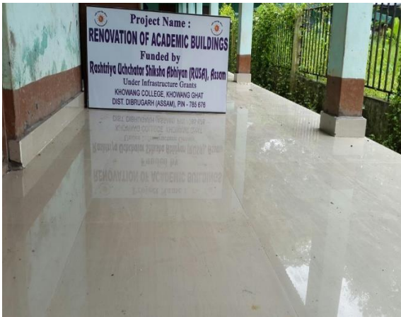
Renovation of Academic Building, Khowang College
