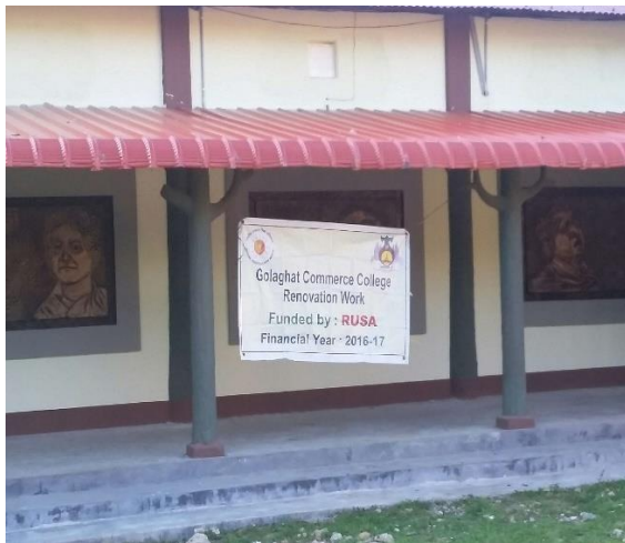
Renovattion Work, Golaghat Commerce College
