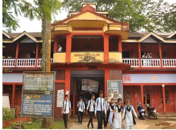
Renovation of Existing Main Building, Karimganj College
