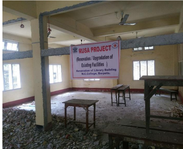
Renovation/Upgradation of Existing Facilities, MC College
