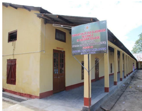
Renovation of Old Classroom Building, Chaiduar College
