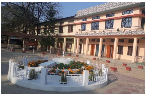
Upgradation of Academic Building of Dhemaji College
