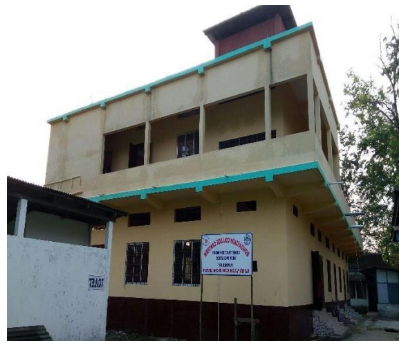
Construction of College Canteen Bongaigaon College
