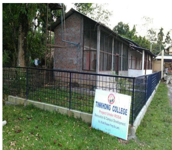
Renovation and Campus Development, Tingkhong College
