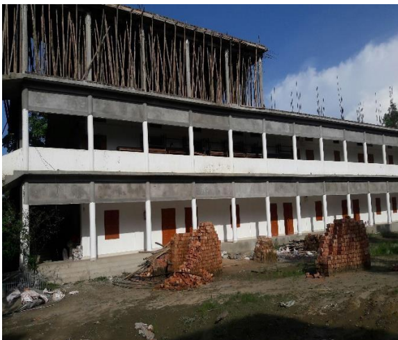
Construction of New Building, N.C. College
