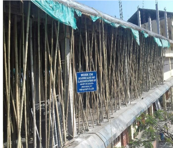
Construction of Academic Building, Pub Kamrup College
