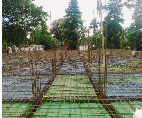
New Construction Work, Dudhnoi College.
