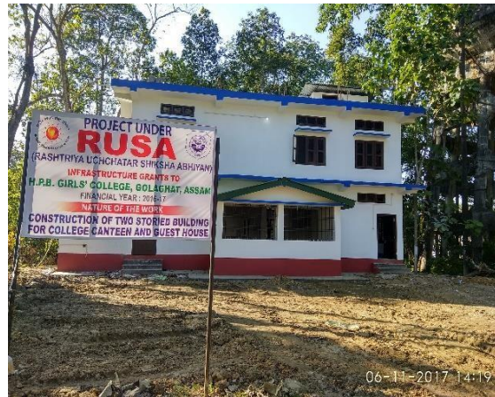
Construction of College Canteen and Guest House, Hemo Prova Borbora Girls' College
