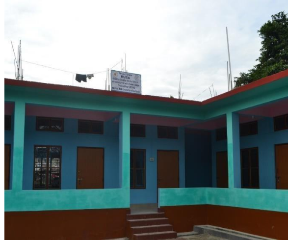
Construction of Boys' Hostel, Sonari College
