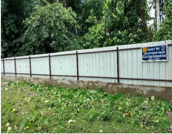
Renovation of Boundary Wall, Kaliabor College
