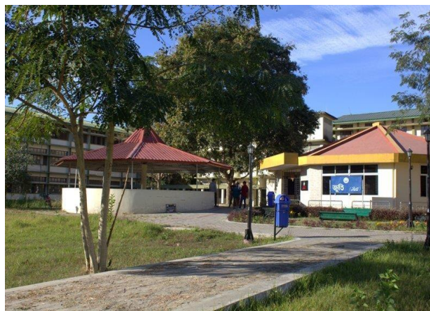
Site Development & Construction of Pathways to the Canteen Building within the campus of Arts Block.
