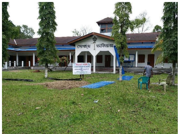
Renovation & Upgradation Work, Gogamukh College
