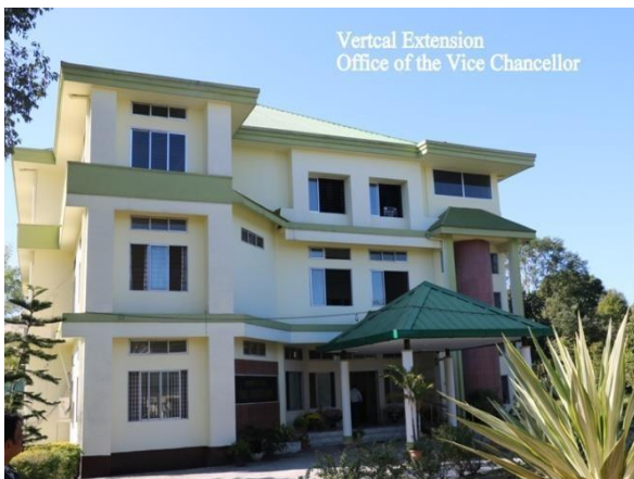
Vertical extension of 2 nd floor of the Vice-Chancellor's Office Building D.U. (Phase-I, Providing Roofing's and finishing of external walls only) (Civil works)
