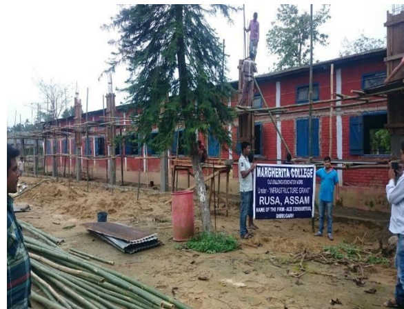
Renovation of Old Building, Margherita College
