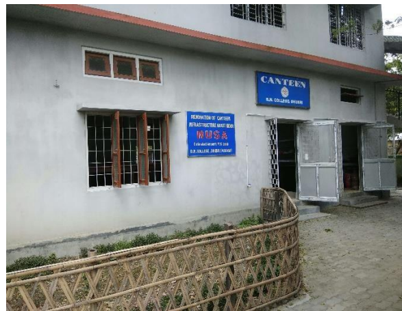
Renovation of Canteen Bhola Nath College
