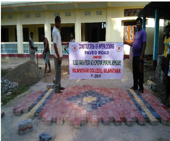
Constrution of Interlocking Paved Road, Silapathar College
